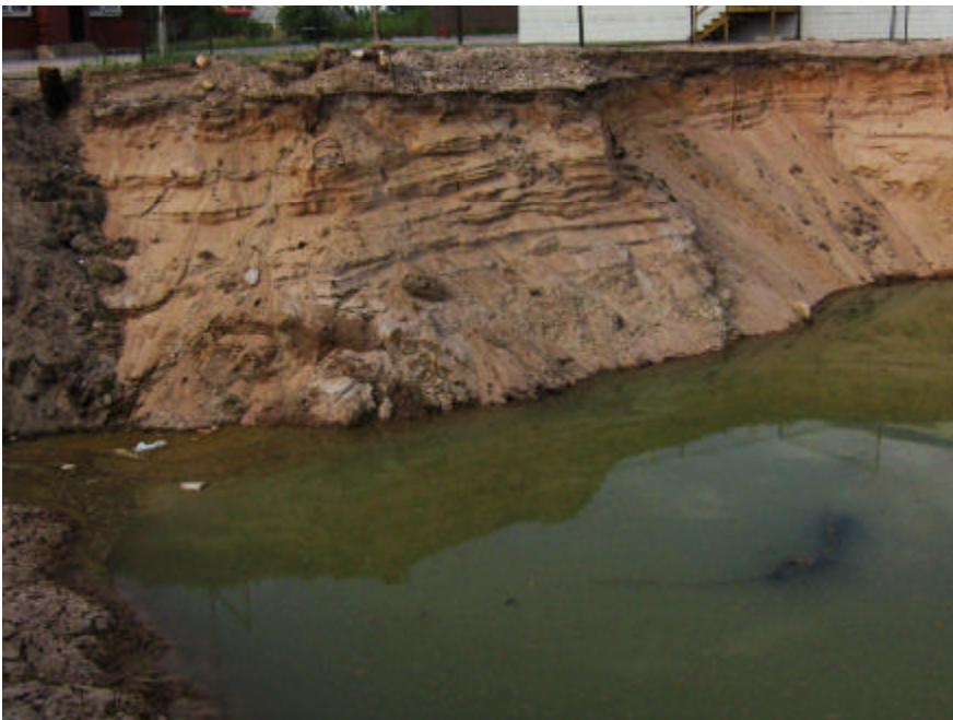
Figure 12. Part of the excavation to remove sands contaminated by diesel fuel in Fort Chipewyan. 2 June 2007.
