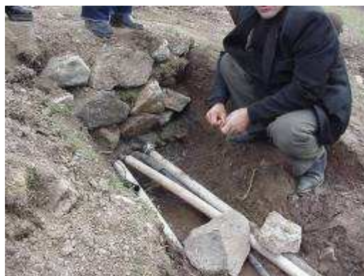
Construction of daily distribution basins.
