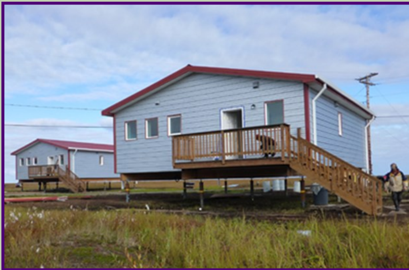
Energy efficient homes in Atmautluak by the Cold Climate Housing Research Center.
