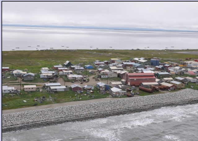
Seawall at Shishmaref (Shorezone).
