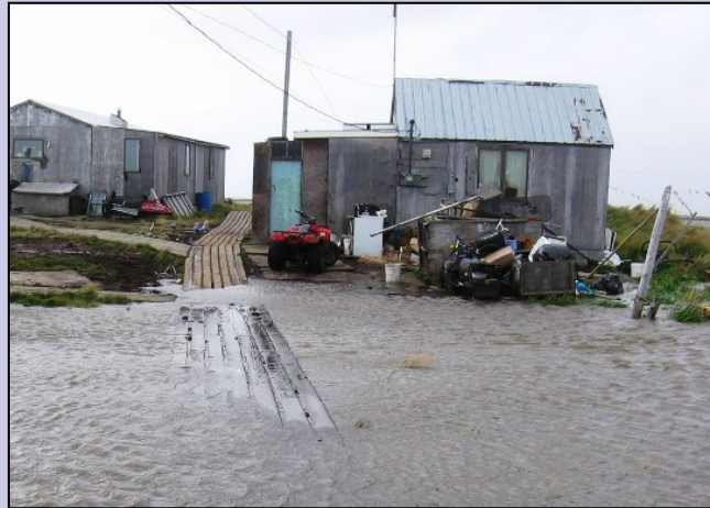
Flooding in Newtok (State of Alaska DCCED DCRA).
