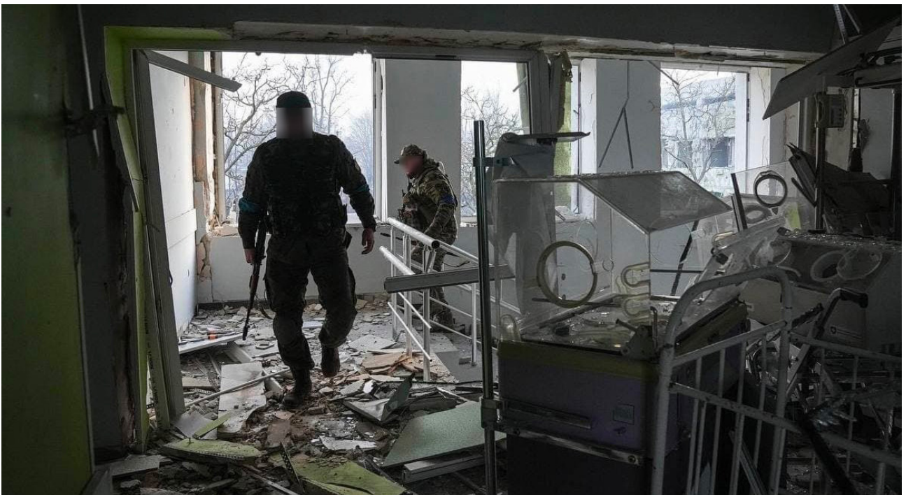
Figure 21: Damage inside the Maternity Ward 3, Myru Avenue, 80. 136
