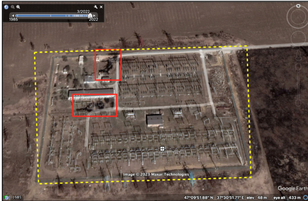
Figure 3: Azovska-220KV Substation, with signs of possible damage. Google Earth Pro (c), Maxar, Image dated March 2022.
