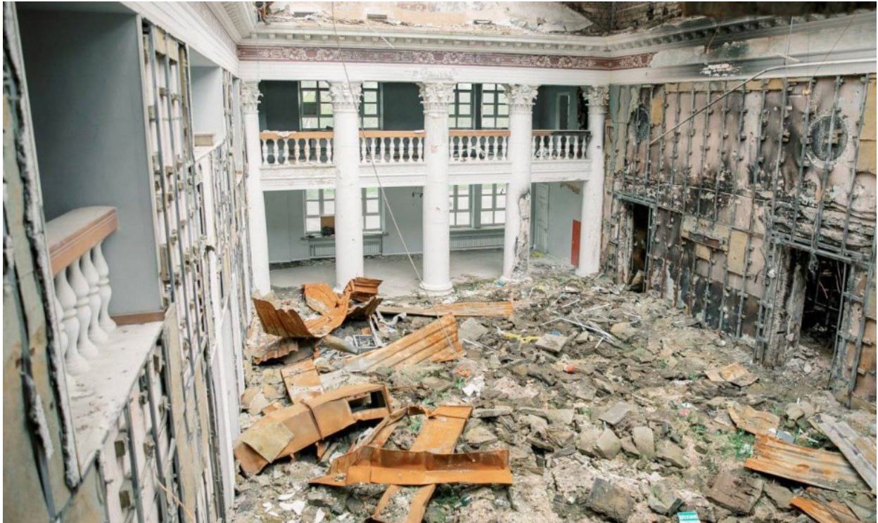
Figure 24: Livoberezhnyi Palace after the attack. Image by Mariupol City Council 165
