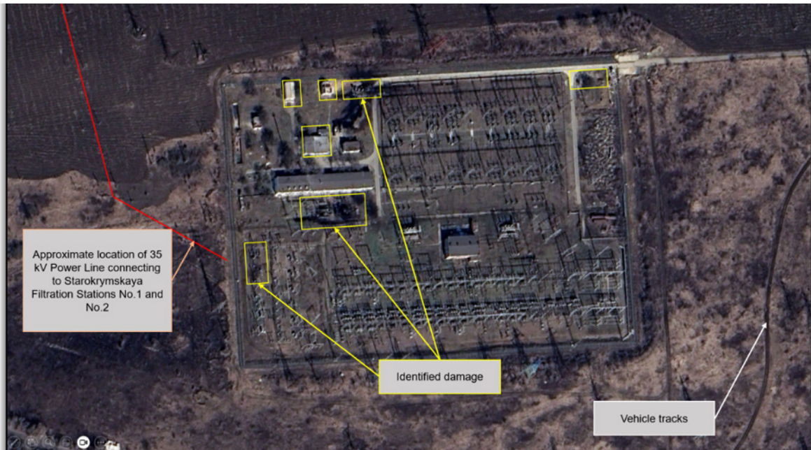
Figure 7: Azovska 220kV Substation. Google Earth Pro (c), Maxar, Image dated 14 March 2022.
