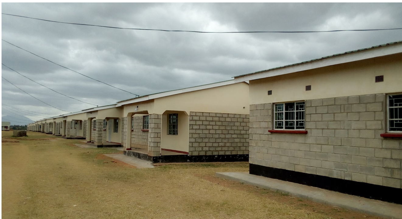
Figure 15: Newly constructed staff houses at Mpyupyu prison.
