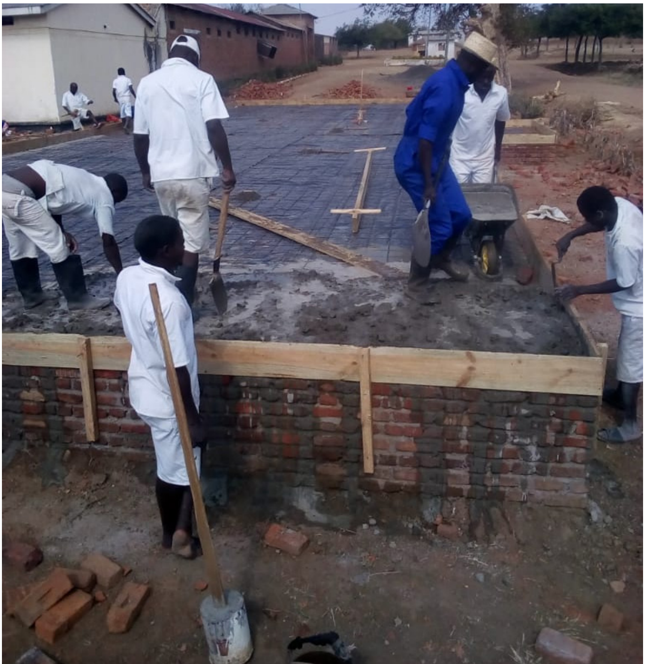
Figure 13: Construction of a cell block at Nkhotakota prison by inmates
