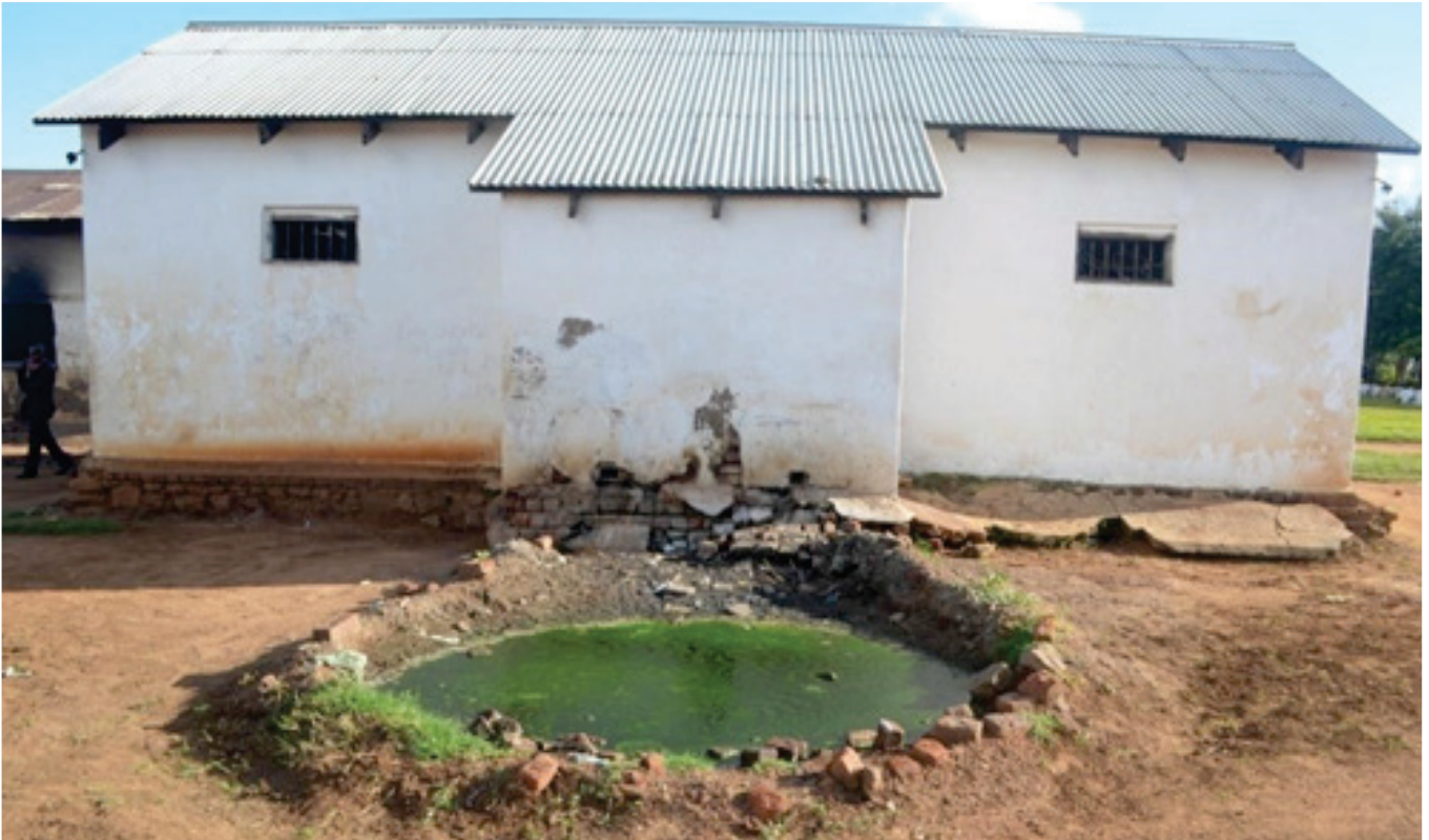
Figure 17: An open ditch containing human excreta behind a cell at Mpyupyu Prison
