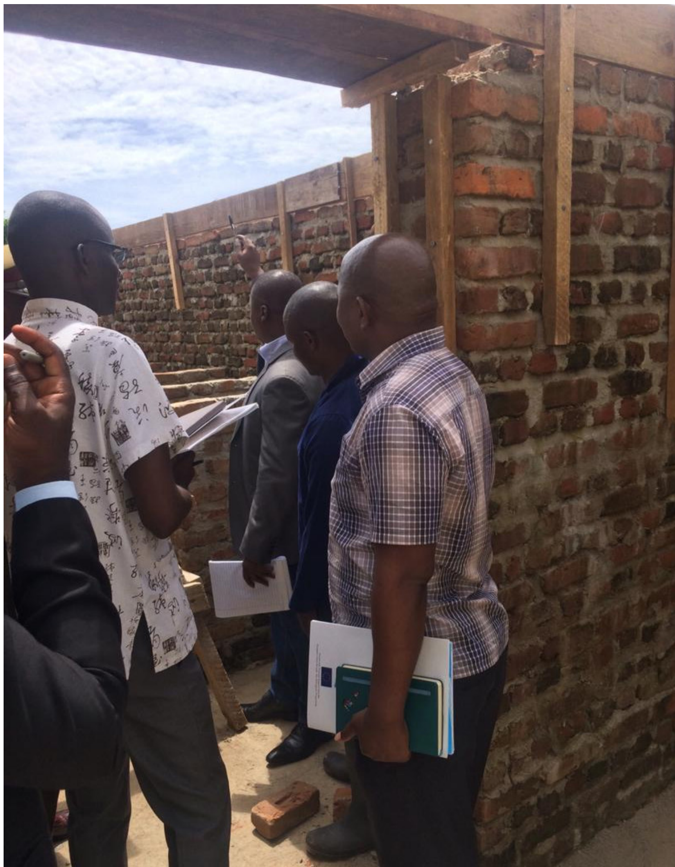
Figure 6a: Inspectors inspecting new cell block at Nkhotakota prison in May 2020.
