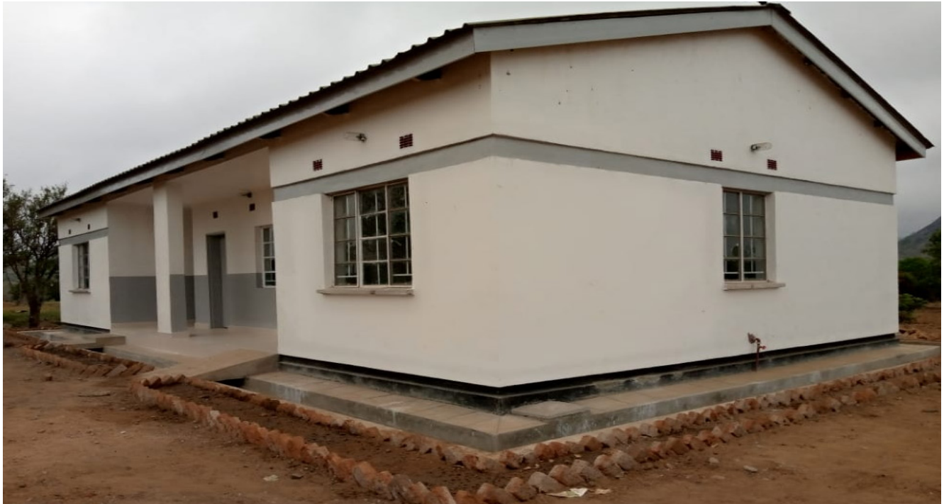
Figure 9: Clinic constructed at Mwanza Prison with support from UNODC.
