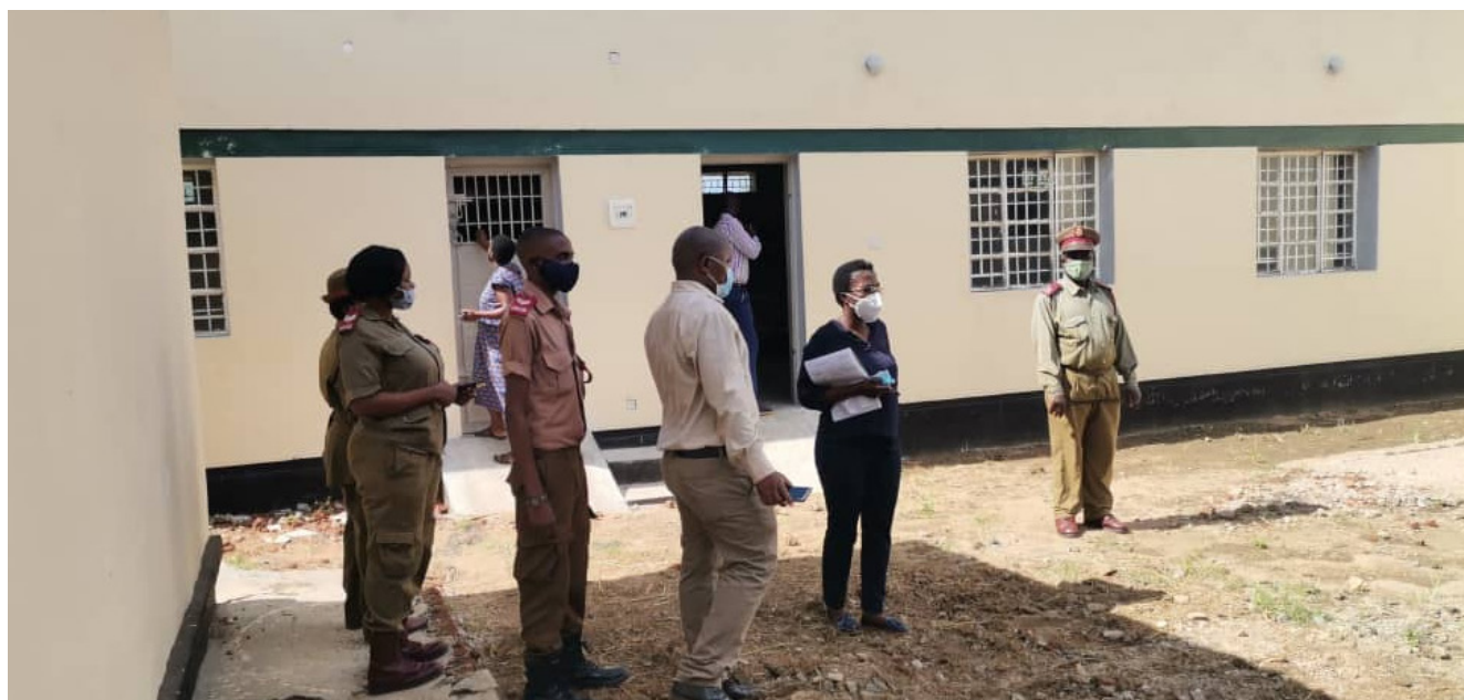
Figure 6b: Inspectors inspecting a newly constructed cell block at Nkhotakota prison during the 2nd wave of COVID-19 in February 2021..
