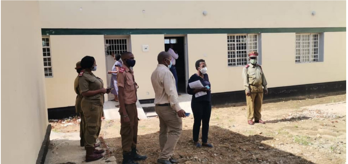
Figure 6b: Inspectors inspecting a newly constructed cell block at Nkhotakota prison during the 2nd wave of COVID-19 in February 2021..
