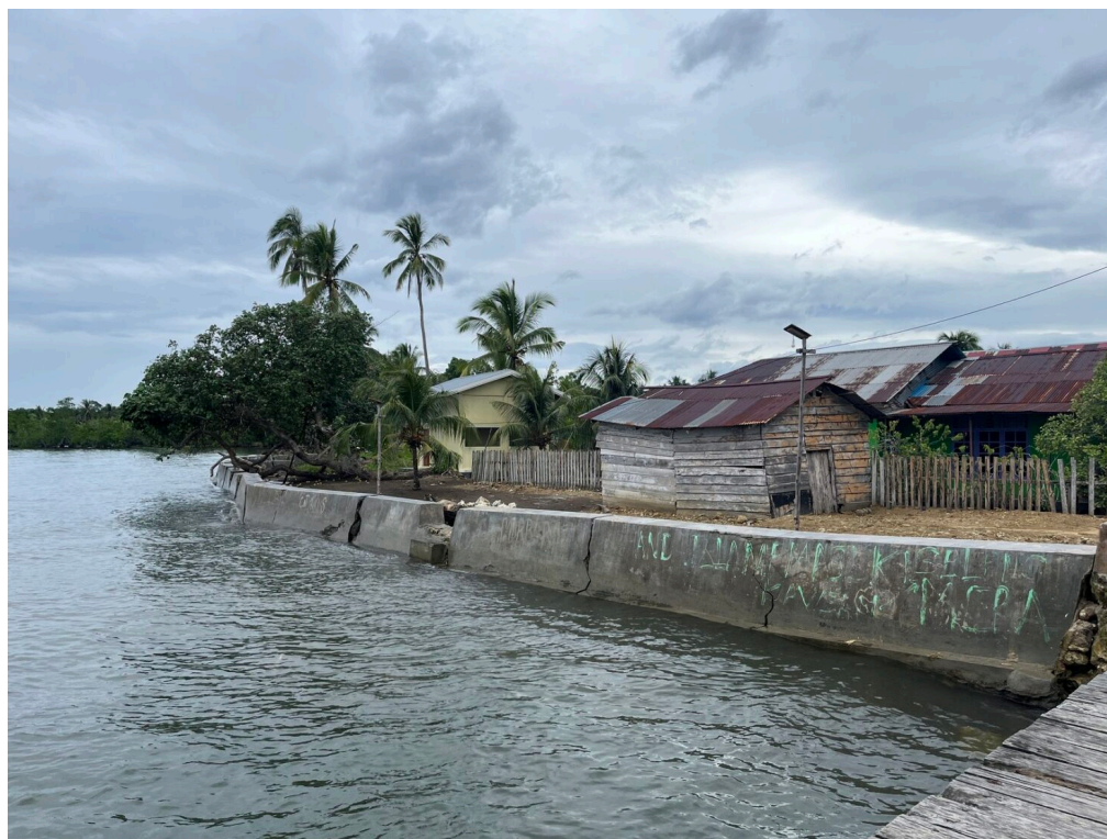
A seawall protecting houses in Waleh, Halmahera from sea level rise, coastal flooding, and extreme weather events.
