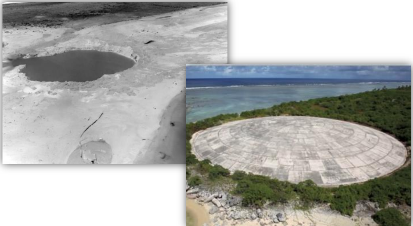
Cactus Crater before (left) and after (right) construction of the Cactus Crater containment structure (i.e., Runit Dome)
