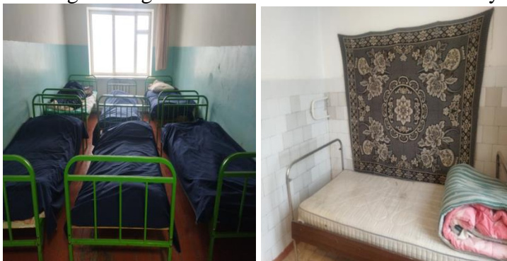
Photo 76. Overcrowded living rooms Photo 77. Room of the isolation ward after renovation
