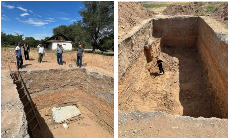
Photos 74, 75. Excavation site on the territory of Tokmok SSI in August 2023
