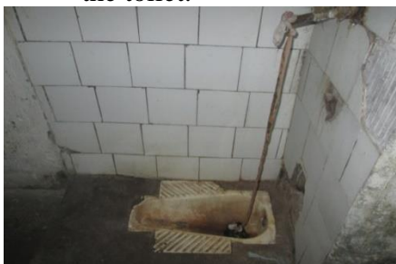
Photos 53, 54. Drinking water faucet is located above the floor sink of the toilet in the PIC cells of Facility No. 3.
