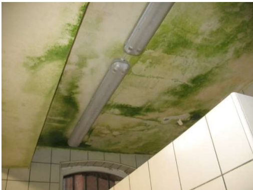
Photograph 17 (Bathroom at Lepoglava Penitentiary)
