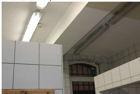
Photograph 18 (Bathroom at Lepoglava Penitentiary after remediation)
