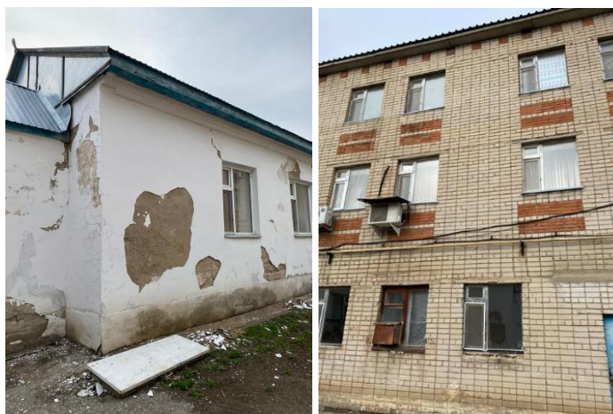
The building of the CSS No. 1 in Aktobe.
