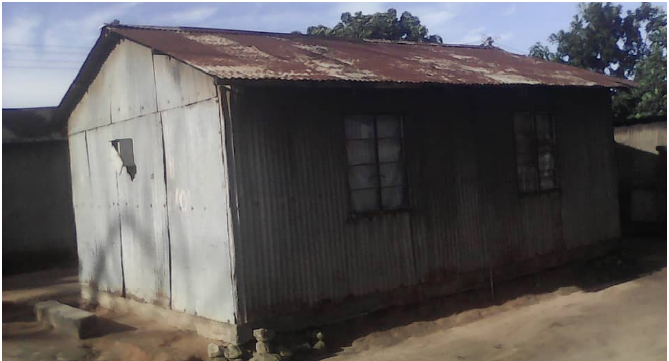
Figure 16: Tin staff house at Mzuzu prison
