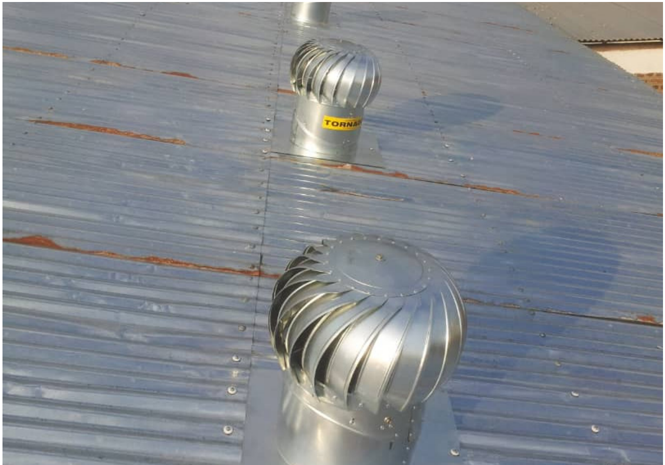
Figure 8b: Whirly birds installed at Chikhwawa prison.
