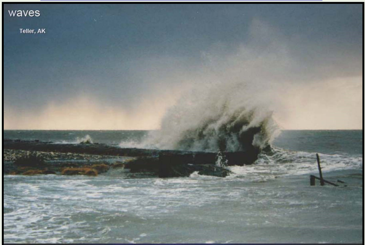
Photo 1: Waves hitting Teller seawall; photo courtesy of David E. Atkinson, UAF, International Arctic Research Center, 2007.
