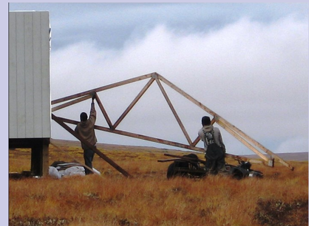
Residents from Newtok building homes at relocation site Mertarvik (Stanley Tom).
