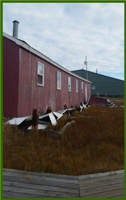
Moravian Church affected by permafrost thawing (Bernice Sallison).
