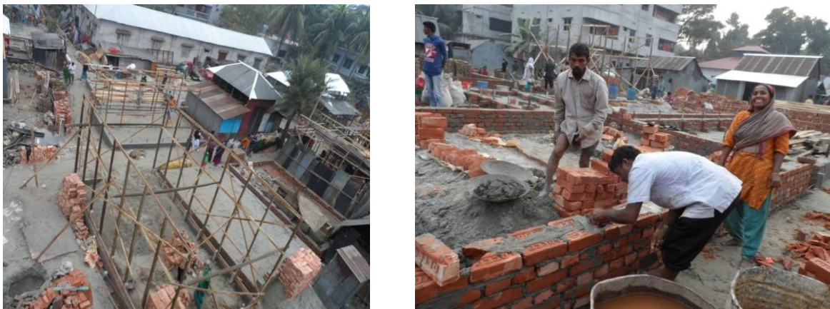
Figure 4.33: Construction works the community people.
