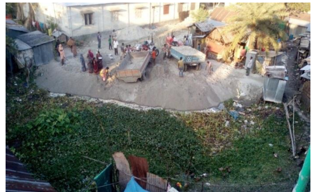
Figure 4.29: Land filling and construction of footpath.
