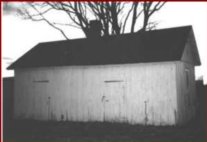
Two Room Slave Quarters Before Demolition
