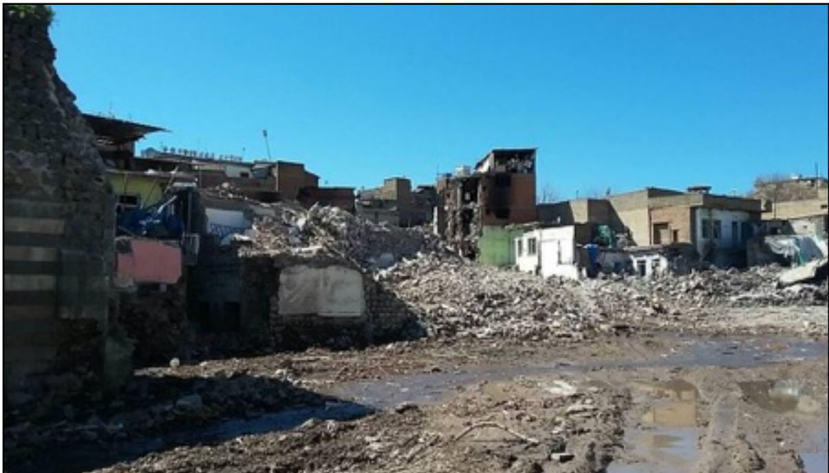
PHOTO 15- DEVASTATION OF HISTORICAL BUILDINGS
