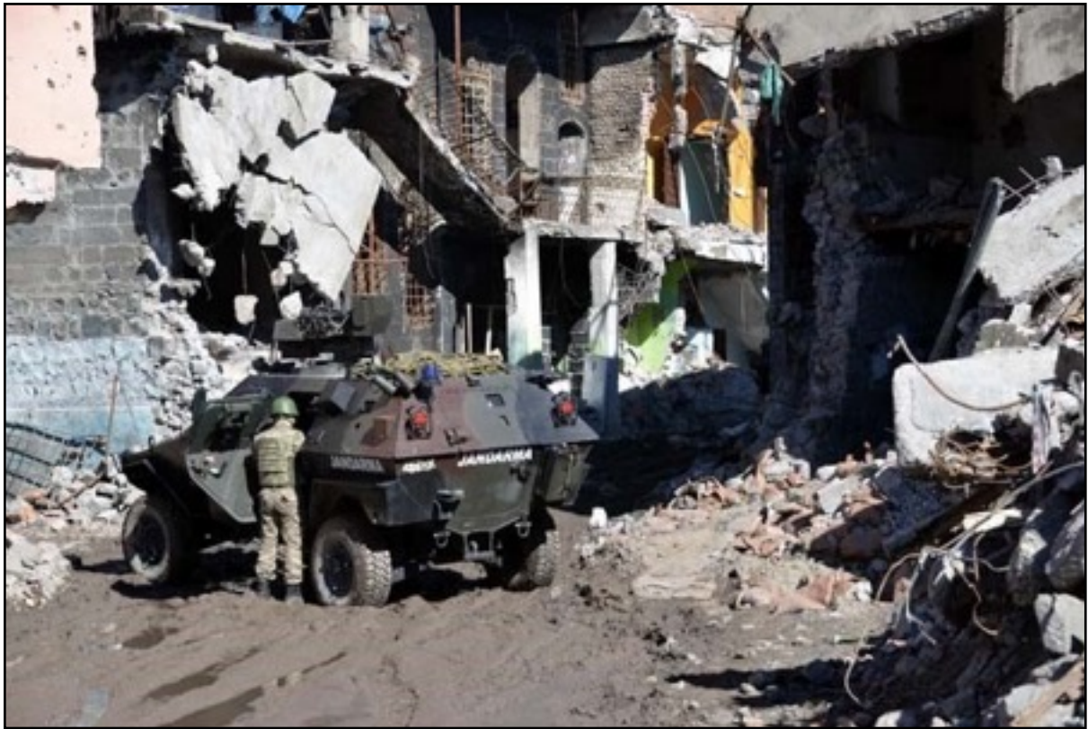
PHOTO 13- DEVASTATION OF HISTORICAL BUILDINGS
