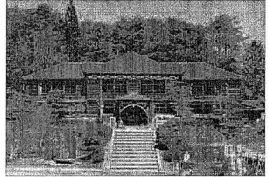
Old Fukiya Elementary School Main Building, designated as an Important Cultural Property by Okayama Prefecture
