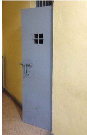
Small window with horizontal bars at the Police Station of the CNP of San Blas district, Madrid
