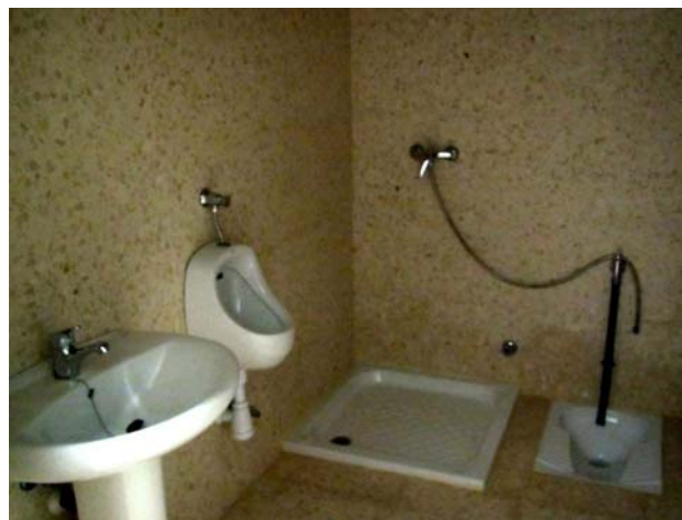
Porcelain toilet appliances at the Station of the GC of Ciudad Real
