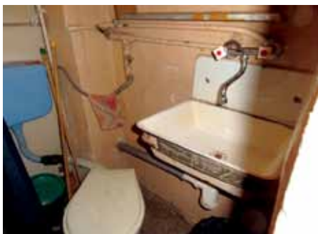
Sanitary area (Pre-Trial Detention Centre in Chojnice)
