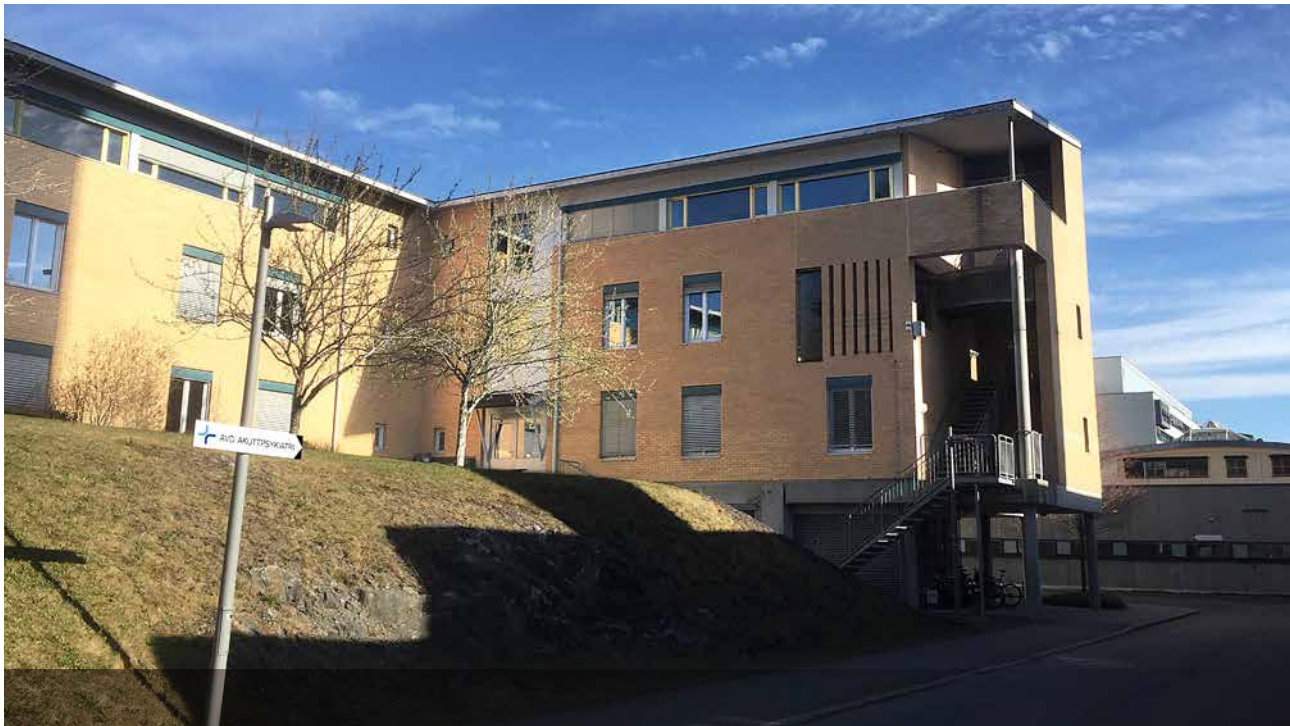
Akershus University Hospital, the emergency psychiatric department
