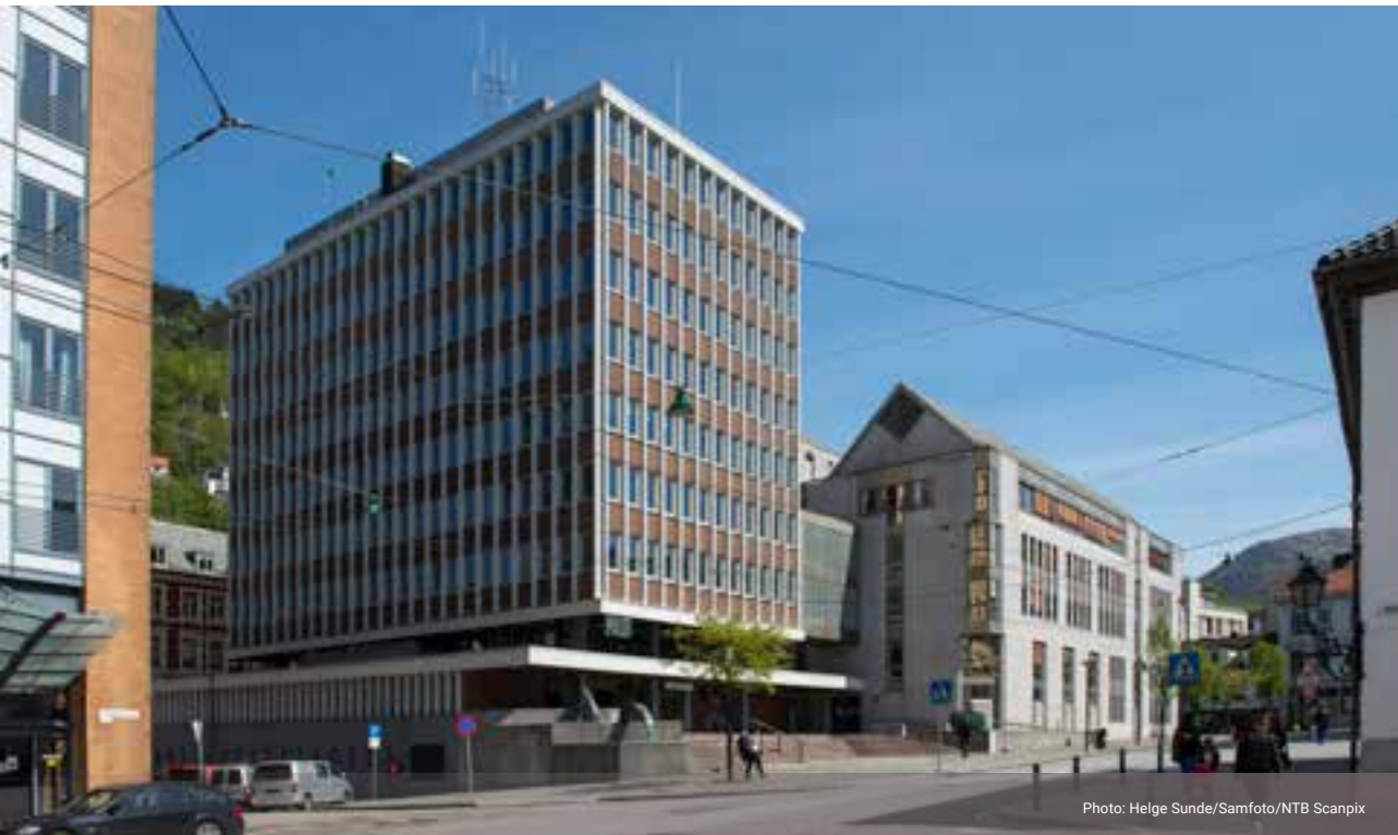
Bergen police custody facility
