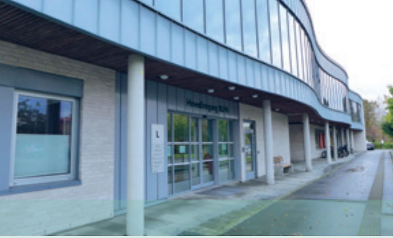
Main entrance to the mental healthcare facility for children and adolescents, Stavanger HF.
