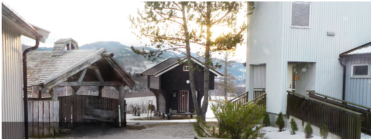
Kvammen emergency institution
