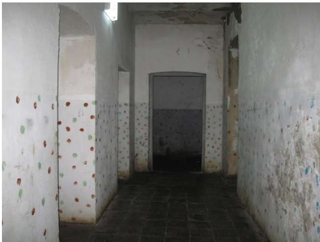
Corridor of Patients accommodation building
