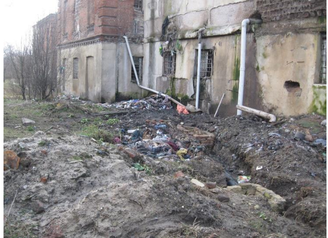
Back side of the Accommodation Building of patients
