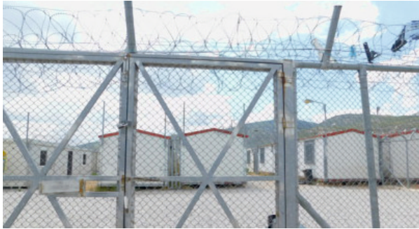
Amygdaleza Pre-removal Detention Center (Attica) - inspection on 18/7/19
