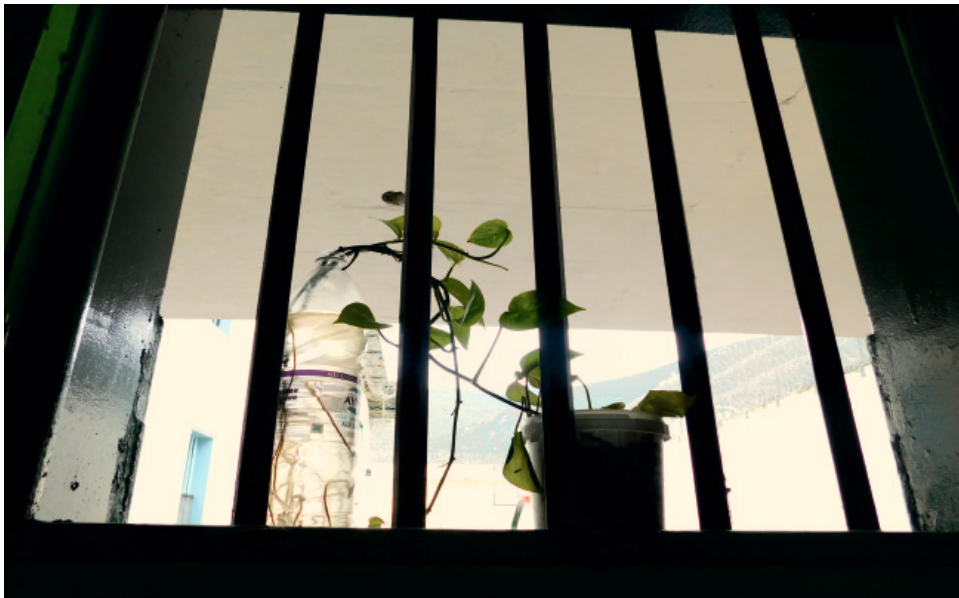
Malandrino detention facility, Fokida - inspection on 25-26/11/19
