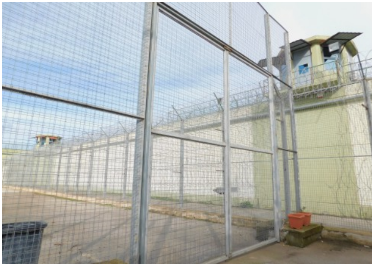
Malandrino detention facility, Fokida - inspection on 25-26/11/19
