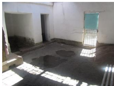
TDF of the IAB of Tokmok City. Exercise yard and toilet.
