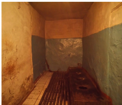
Photo #4. Toilet in the men's unit
