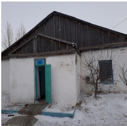
Photo #1. "Main" entrance to EK PH in Novo-Kanayka
