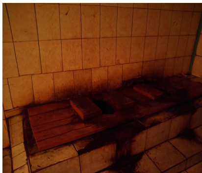
Photo #3. Toilet in the women's unit
