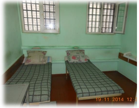
Windows with vent panes allowing for ventilation
