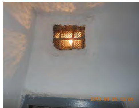
A cell for temporarily detained personnel at Mykolayiv territorial subdivision of PSAFU
