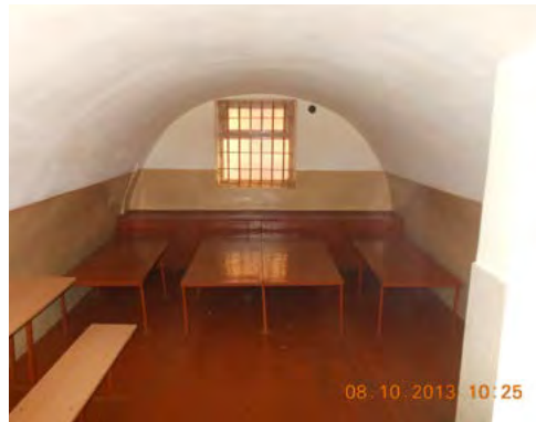
Temporary holding facility in Chernivtsy Region (the distance between the floor and the ceiling is less than 2.5 m)
