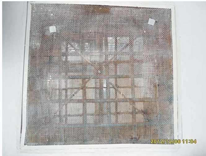
Photo: a window in the temporary holding facility of Volnovakha District Unit, MIA Main Department in Donetsk Region
