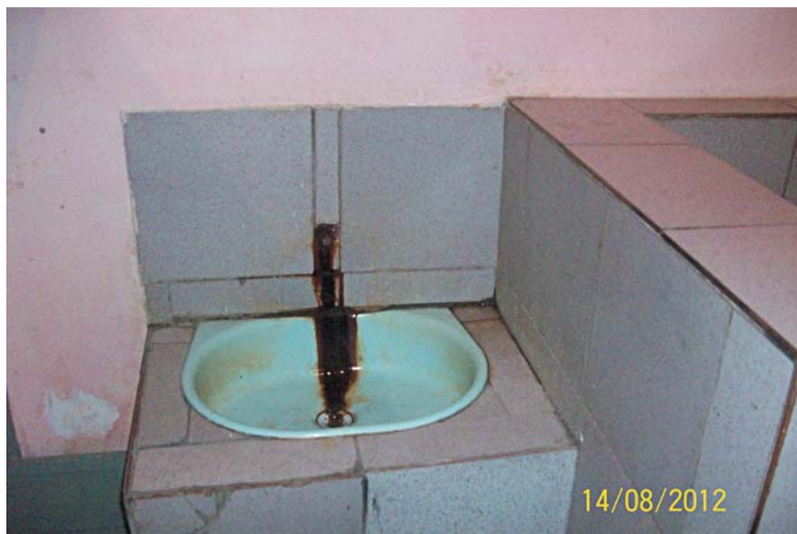
Photo: absence of faucet at the special reception center for persons under administrative arrest, MIA Department of Khmelnytsky Region
