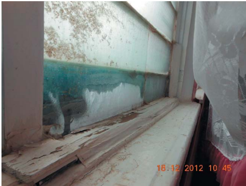
Photo: hoarfrost on the corridor windows at Komyshevaha social rehabilitation and general education school, Zaporizhzhya Region
