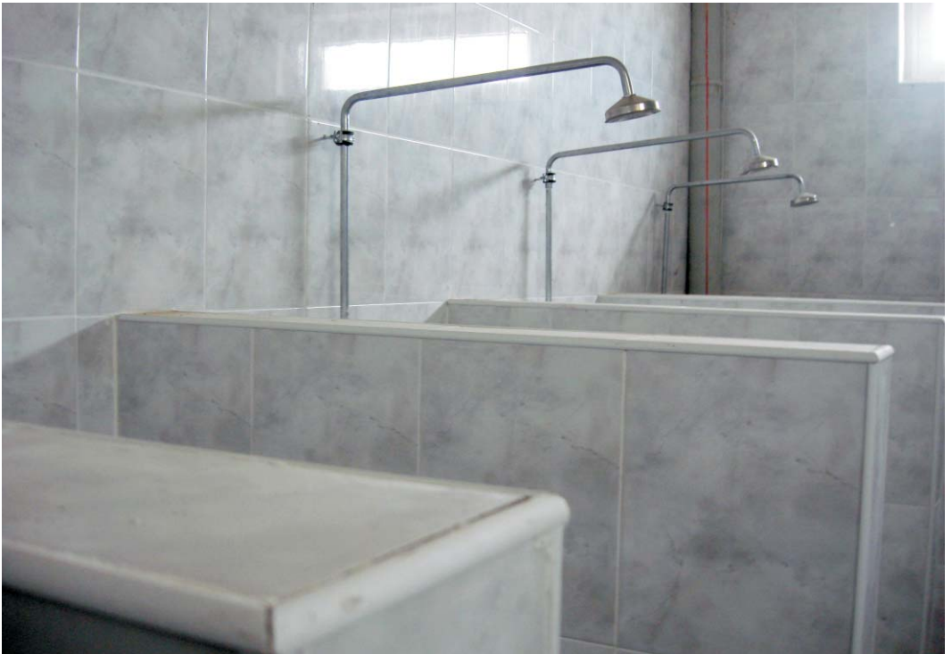
Photo 36. ME Open Special Correctional Institution for Boys. New bathroom.
