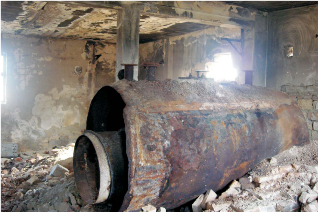
Photo 33. ME Open Special Correctional Institution for Boys. Old boiler room.
