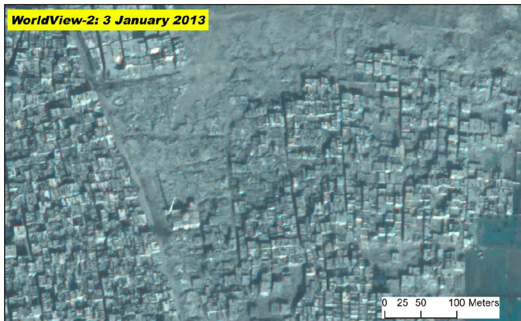
At top, the area of Damascus known as Tadamon, as it appeared on 22 August 2011. By 3 January 2013, at bottom, large portions of the neighborhood had been razed. UNOSAT analysis estimates that almost 1,000 structures in the area were destroyed by demolition. Images copyright 2013 DigitalGlobe; image from 22 August 2011 obtained from Google Earth.
