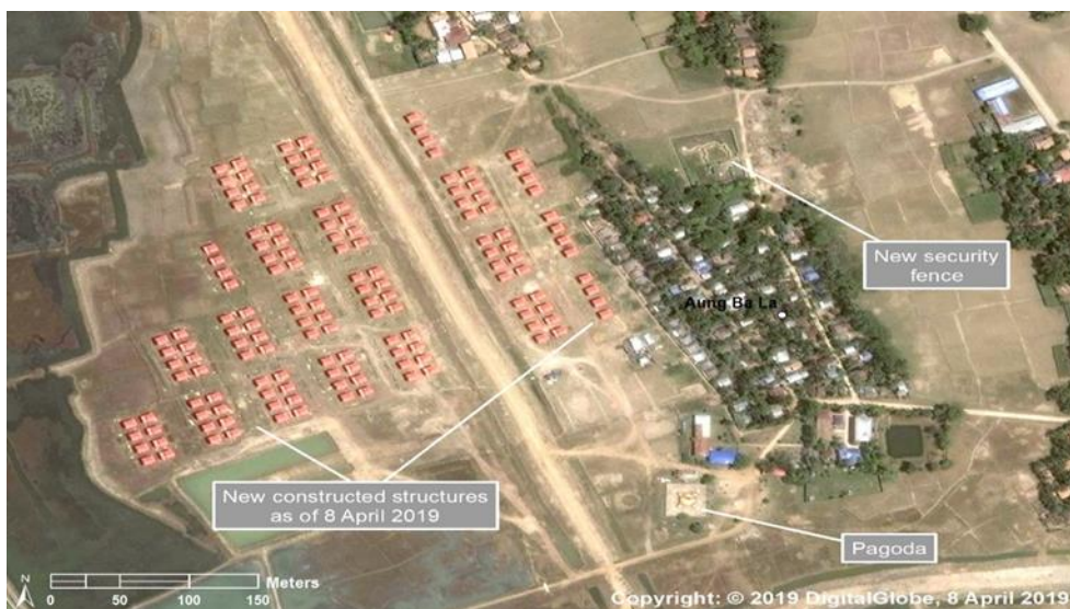
Image of Aung Ba La, Shwe Zar Kat Pa Kaung village tract, Maungdaw Township as of 8 April 2019 showing the completion of new structures near the village
