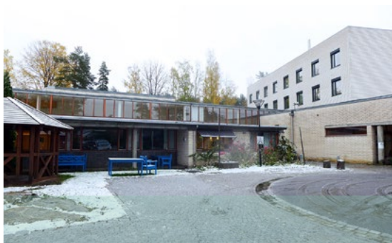
Høyås Residential and Rehabilitation Centre, Nordre Follo Municipality. Photo: NPM
