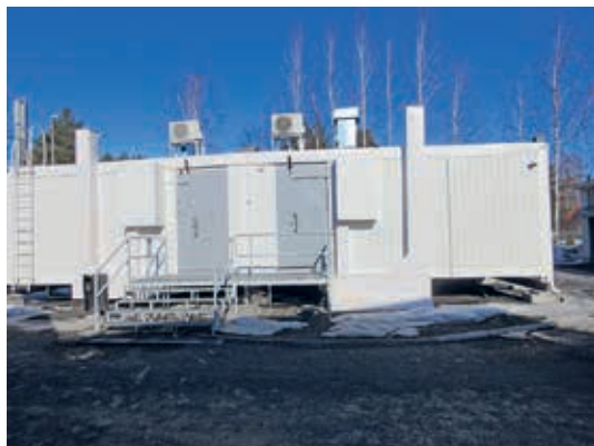
Containers have been used to form the cells in the temporary module prison at the police station.
